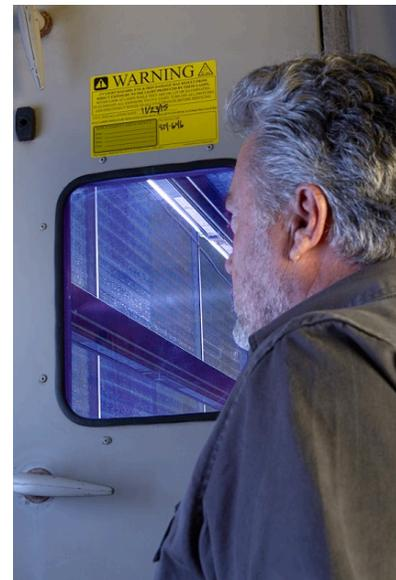
Jim Edson of NUVView Environmental, a distributor for UV Resources, inspects High-output DEF (Double-Ended Fixture) UV-C fixtures installed in one of LAX's more than 200 air handlers. The UV-C energy helped boost airflow by 15 percent.
