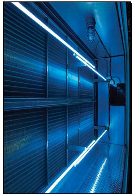
**The RLM Xtreme fixtureless UV-C lamp system from UV Resources creates a more energy-efficient HVAC system that doesn't have to waste energy to move air.**
